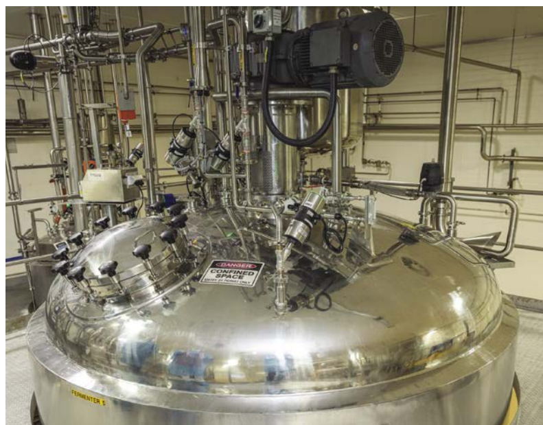
DFS Fermentation tank with pH and temperature monitoring
